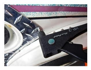
Insert the pop rivet into the drilled holes, press hard against the Diamond Plate Corner and squeeze the handles of the pop rivet gun together.
